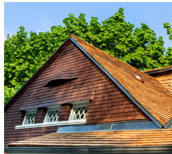
Close-up from the south of the steeply pitched, cross gable roof clad in wood shingles (L) Close-up of the corbeled oriel window on the south façade of the second storey of the gardener's cottage (R).
