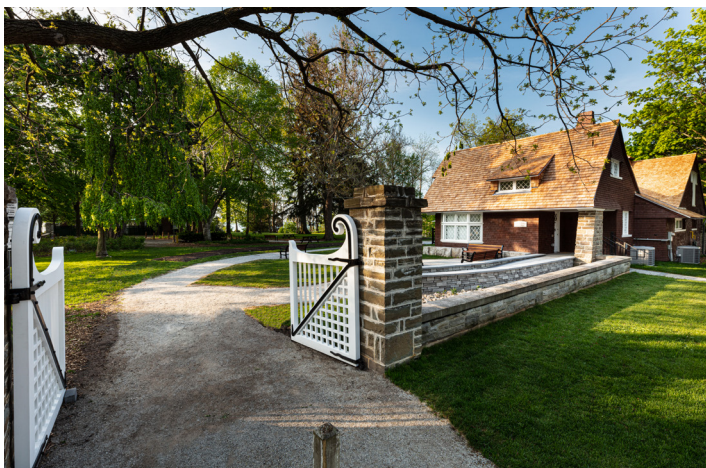
The ornamental wooden gate at King Street, a significant landscape feature, leads to the Coach House's east entrance. A barrier-free entrance was created by rebuilding the existing porch 46-cm higher with the entrance preceded by a gently sloping path over an archaeological zone that brings the visitor to the level of the door threshold.
