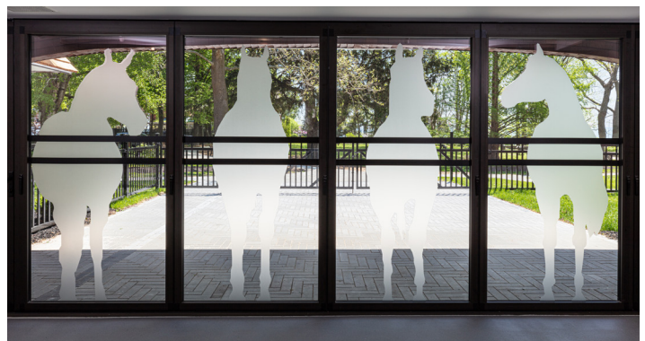
The south façade's barn doors added during a 1997 renovation were replaced with a new operable glass wall panel system with a film graphic depicting horses.
