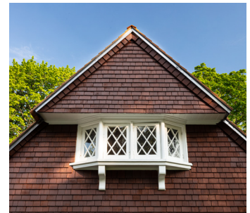
Close-up from the south of the steeply pitched, cross gable roof clad in wood shingles (L) Close-up of the corbeled oriel window on the south façade of the second storey of the gardener's cottage (R).
